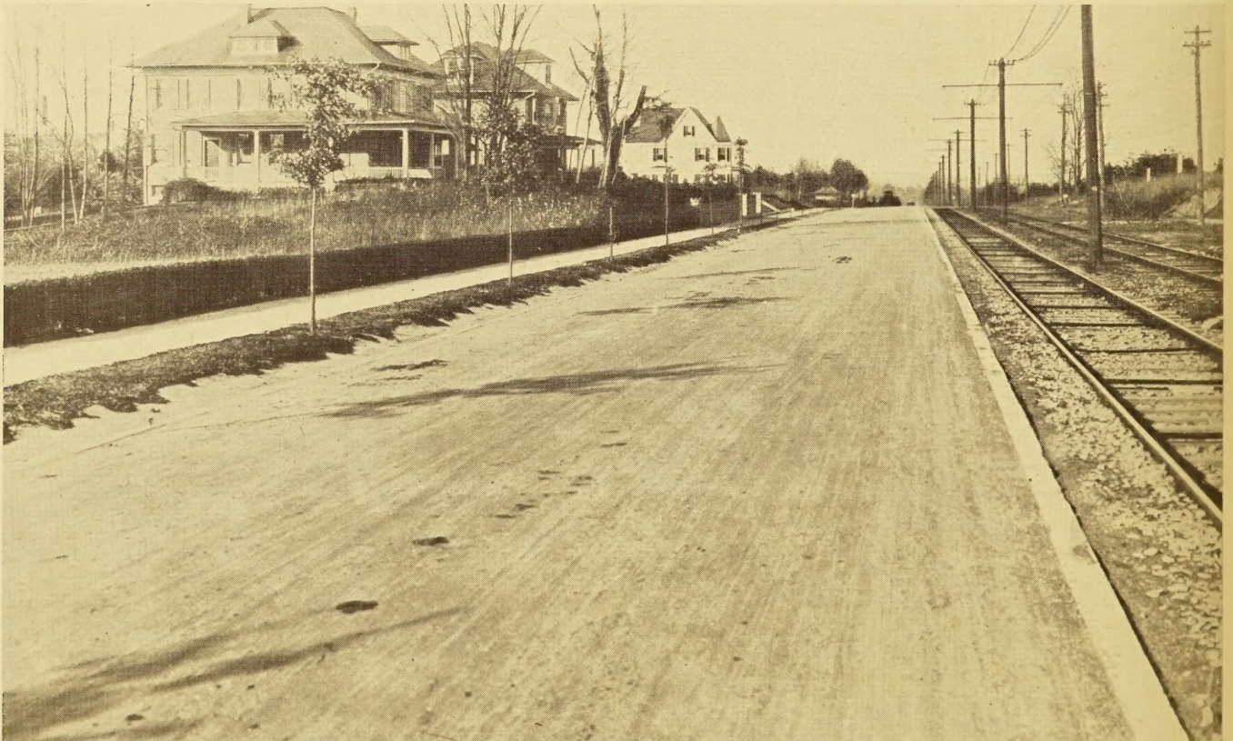
CONDITION OF BITUMINOUS CONCRETE SURFACE AFTER ONE YEAR OF SERVICE, DECEMBER, 1913
